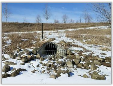
Small trees and other woody growth, as well as sediment and other debris can damage the structures or block the free flow of stormwater.
